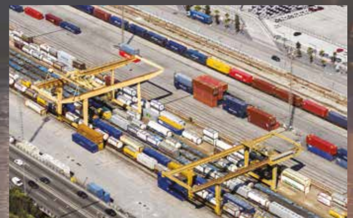
Rail-Mounted Gantry (RMG) Crane
